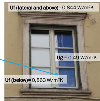
The question of integration of shading systems in the window/glazing system from conservation point of view strongly depends on the building, the window, the type and colour of the shading. In the monumental school in Innsbruck has been applied a lamellas redirecting system (mid pane) which fits very well into the cavity of a box type window with a wide space between the glazing. It is not applicable in coupled windows, because of the wide lamellas.
