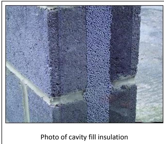
External insulation (8.2) may also be required to meet the U-value targets. It is important to note that external insulation applied to a cavity wall will not perform well as there is still a ventilated void of cold air on the wrong side of the external insulation. It is therefore an essential first step to inject a cavity wall with insulation before external insulation is installed.
