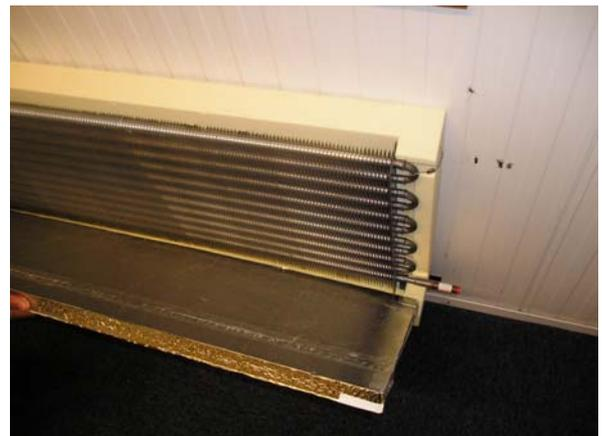
8. vacuum insulation sheet between heat exchanger and convector chimney
