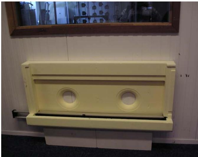
10. Insulation package and self regulating valve
