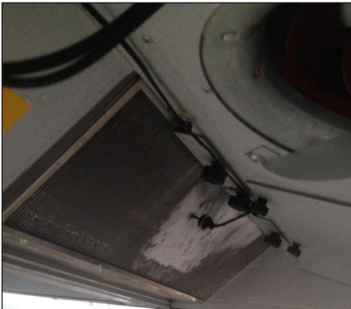
Figure 9: Photos of the counter flow heat exchanger shortly after test drive 2
