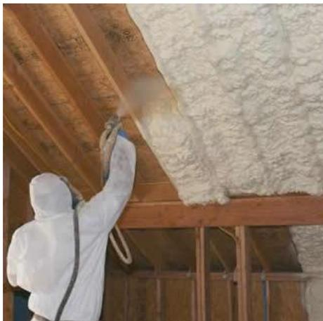
Figure 6 : Foam thermal insulation technology
