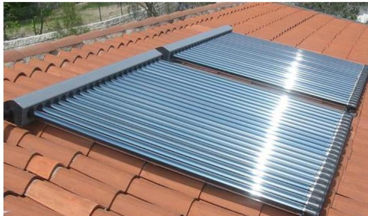
**Figure 39 : Vacuum tube solar water collector**
