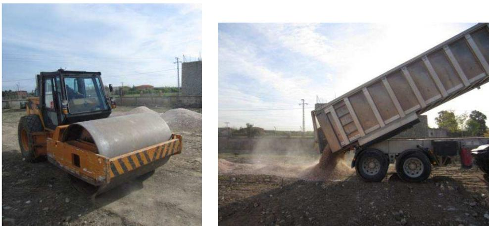
**Figure 6** Ground preparation works.
