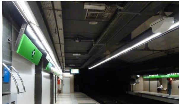
Figure 25. STI Lamp configuration 1x36 + 1x36.
