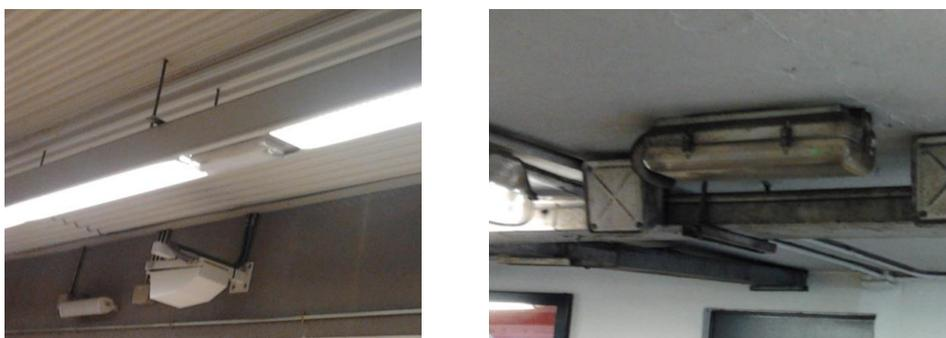
Figure 27. Different configurations of emergency lighting in PdG-L3.
