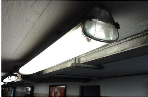
Figure 24. Carandini 2x36W lamp in L3 PdG.
